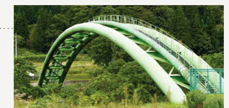
△ Niigata-Sendai Gas Pipeline
