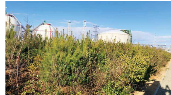
△ Planting trees of native species at the Fukushima Natural Gas Power Plant
