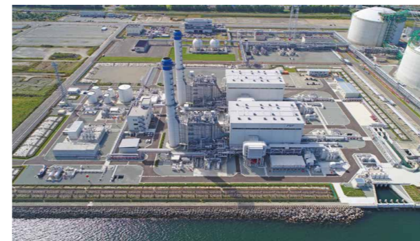
△ Fukushima Natural Gas Power Plant (Fukushima Gas Power Co., Ltd.)
