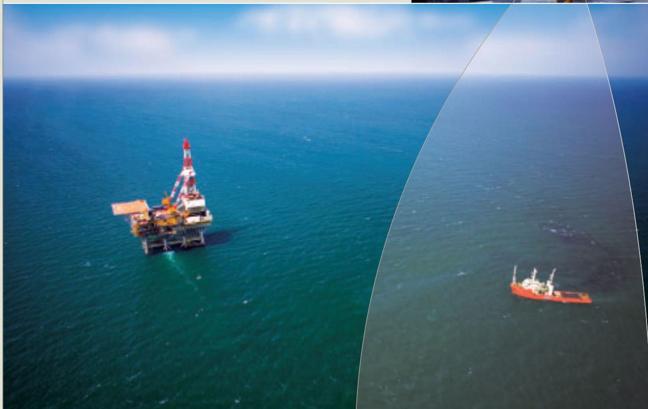
Iwafuneoki oil and gas field platform (Niigata)
