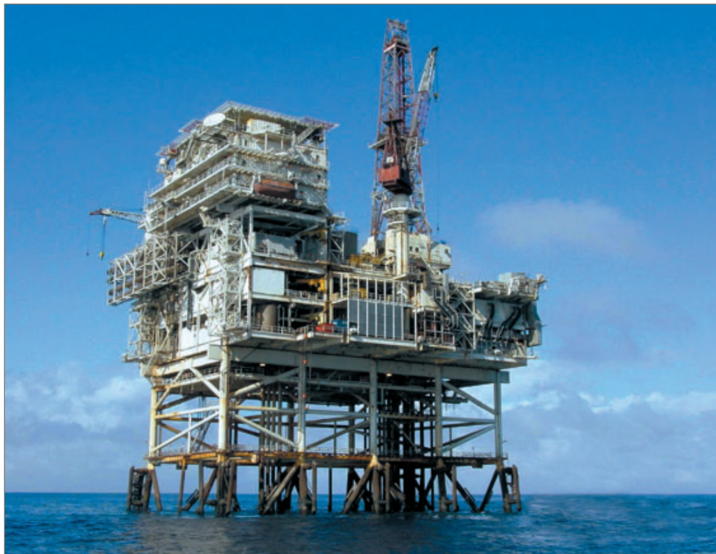
A Platform in the Lufeng 13-1 Oil Field (China)
