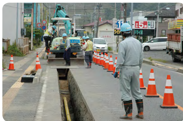
Gas pipeline construction
