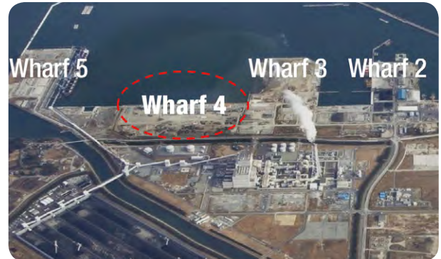
Land designated for the construction of the terminal (Shinchi Town, Fukushima Prefecture)
