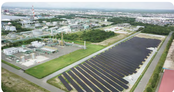
Hokkaido District Office's mega-solar power plant site
