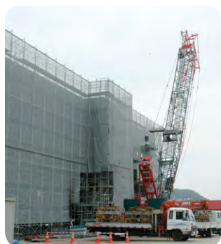
Fukushima Prefectural housing under construction
