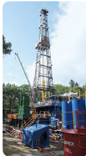
Drilling rig at geothermal site
