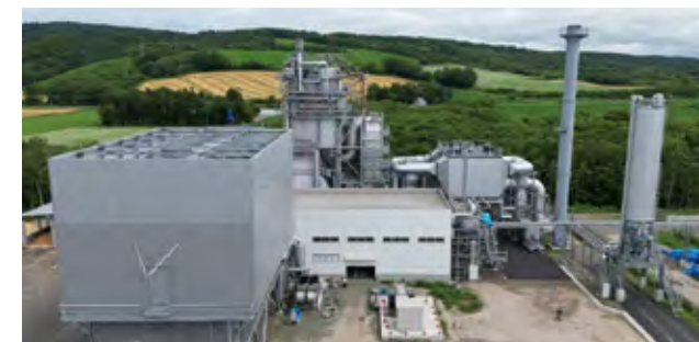
Abashiri Biomass 2nd Power Plant (under construction) in Hokkaido
