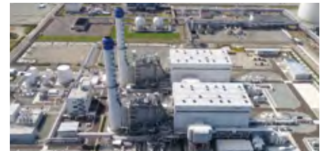
Fukushima Natural Gas Power Plant of Fukushima Gas Power Co., Ltd.
