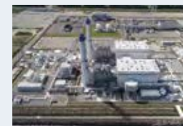
Fukushima Natural Gas Power Plant of Fukushima Gas Power Co., Ltd.
