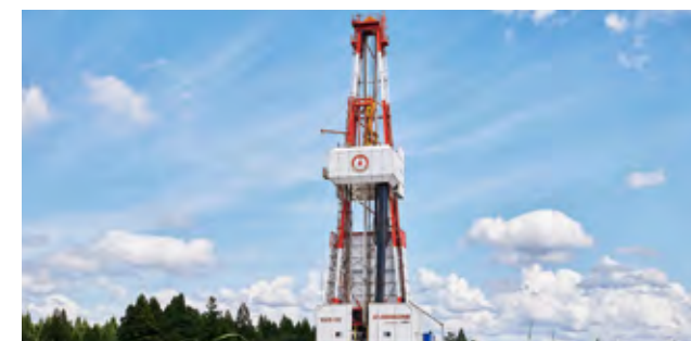
Drilling work site at Katakai Gas Field in Niigata Prefecture
