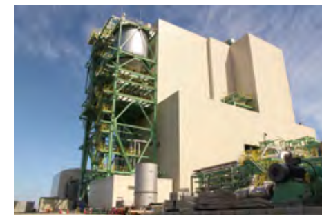
Ehime Prefecture Ozu Biomass Power Plant
