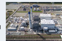
Fukushima Natural Gas Power Plant of Fukushima Gas Power Co., Ltd.
