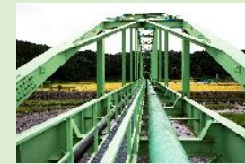
High pressure gas pipelines construction and operation
